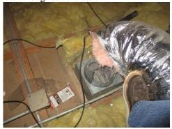
34. Damaged and separated metal ducts throughout the attic.
