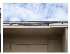
8. Missing head flashing above the protruding exterior trim.
