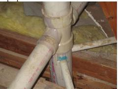
39. Dielectric connections between the copper return lines on the HVAC system and the galvanized hanger strap and the galvanized metal ducts.
