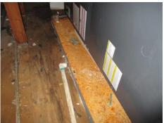
36. Missing insulation on the primary condensate drain lines throughout the attic.
