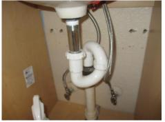
45. Improper drain lines and missing P traps installed under some of the bathroom lavatories.
