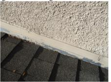
4. Improper termination of the flashings behind the stucco cladding at the roof to wall transitions.
