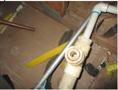
38. Improper termination of the condensate drain lines into un-trapped sewer lines.
