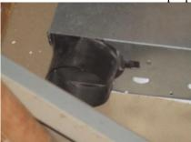
43. Insulation missing from some of the copper supply piping in the attic.
