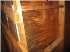
11. Damaged sheathing on the gable ends from the improper termination of the flashing behind the cladding at the roof to wall transitions.
